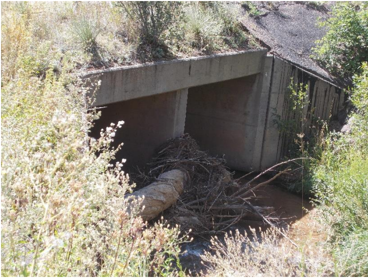
View of structure I-17-X.
